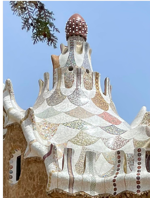
Figure 2: Trencadis tilework from Antoni Gaudí, Park Güell, Barcelona, 1904. Photo by the author.
